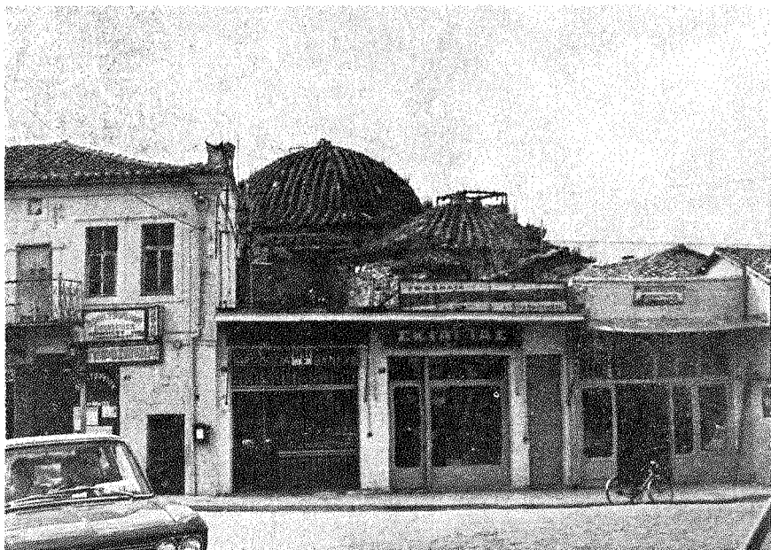
1. Komotini, Ghazi Evrenos Imaret, built-in between shops.
